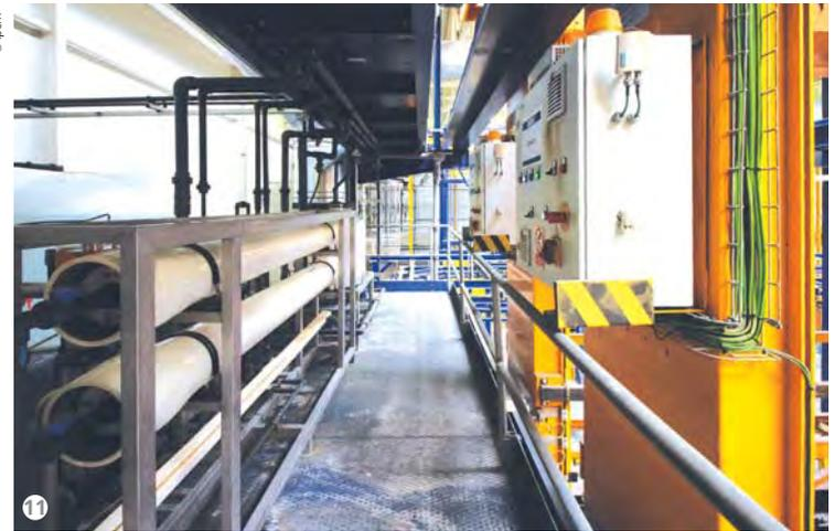
Figure 11: The demineralised water production unit.
